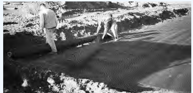
Filter fabric with geogrid placed on top
