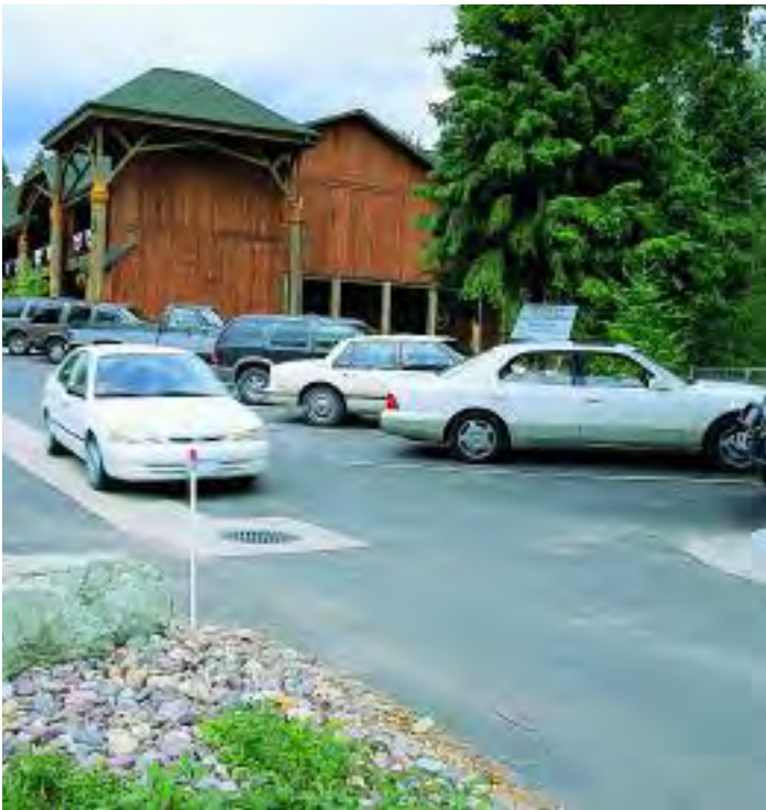
Above: Two views of a completed RS³ install under a parking lot in Big Fork, MT. Parking lot and off-street bays for approximately 48 cars, drains into a 26,250-gallon Rainstore³ stormwater detention structure. Diagonal parking is graded toward the center concrete strip, which drains toward the catch basin.
