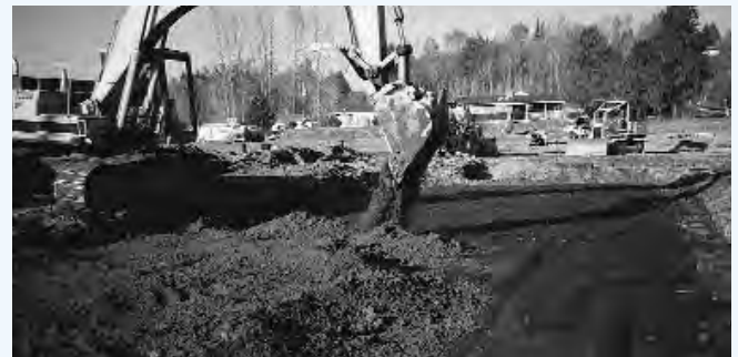
Backfill with roadbase prior to operating heavy machinery on Rainstore 3 units
